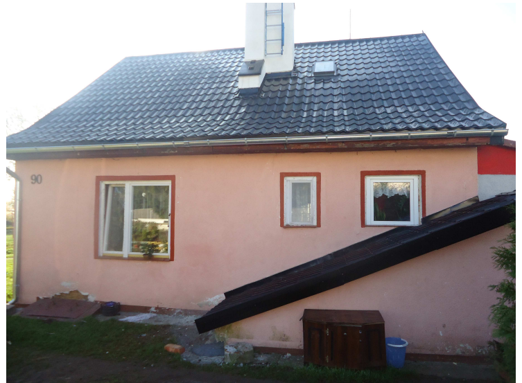
Broczyno 90, remont dachu
