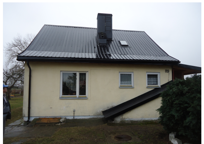
Broczyno 89, remont dachu
